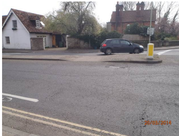
Photograph 2: Splitter island on Ock Street approach
